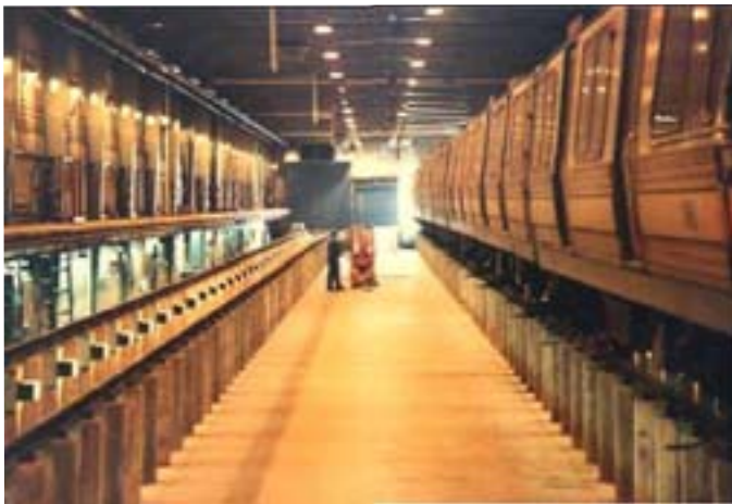
PATH Elevated Rail Facility, Jersey City, NJ
